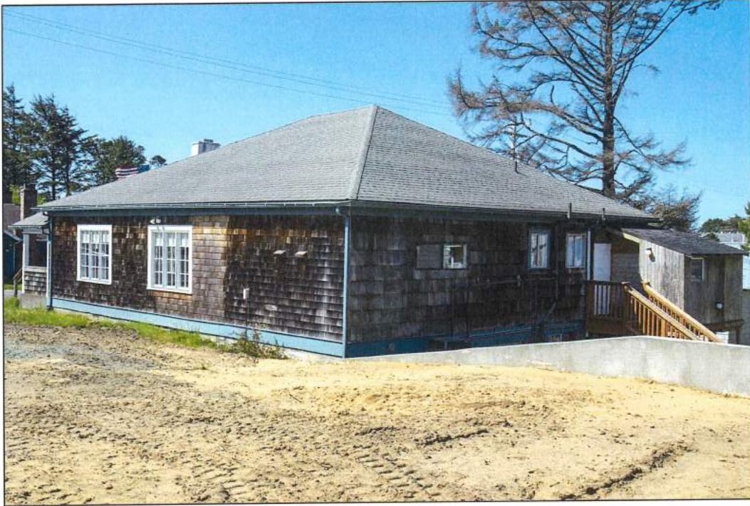
Photo 3 of 15. East and north facades, looking southwest
