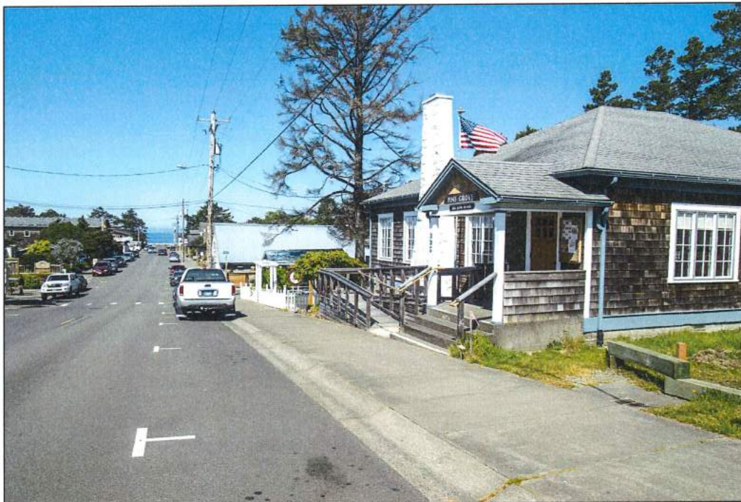
Photo 1 of 15: The building as it sits on Laneda Avenue, looking west
