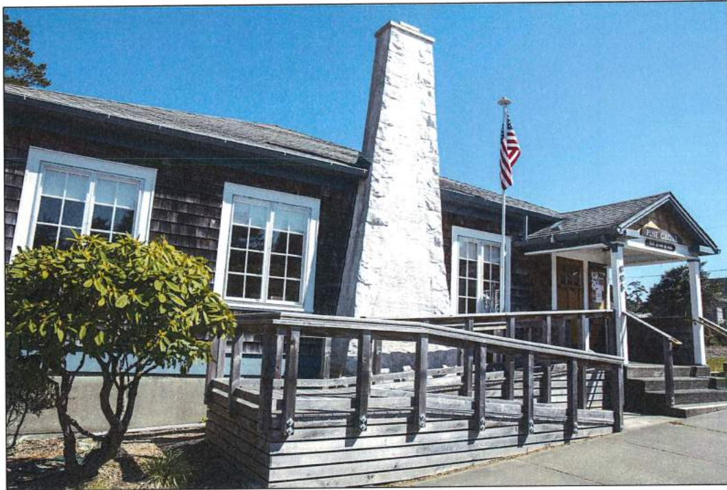
Photo 4 of 15. Front, north façade, including ADA ramp and chimney, looking northeast
